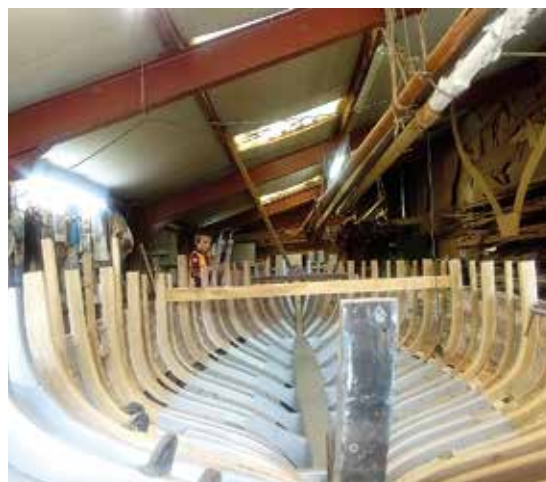
Severn undergoing restoration.
