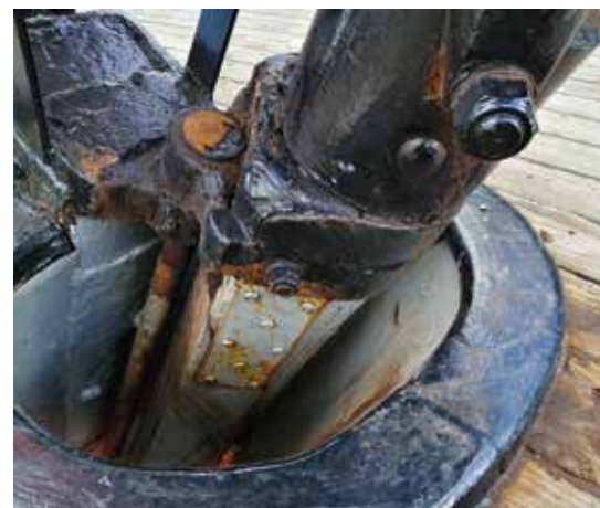
Rudder and tunnel before the work. Photo courtesy of Iain Hunter and Tony Bridle.
