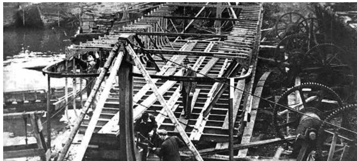
A dumb barge, built to the lines of a Mersey Flat, takes shape on the older patent slipway at Castlerock Yard. This slipway was destroyed by the building of the road bridge to Widnes, and replaced by one further east – Photo from the Mersey Flat Oakdale Facebook page.
