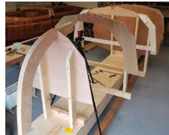
Stem and Bulkheads. Photo by Keith Mcllwain.
