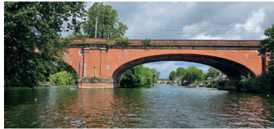
Brunel's Maidenhead bridge - still the flattest long brick arch in the world.
