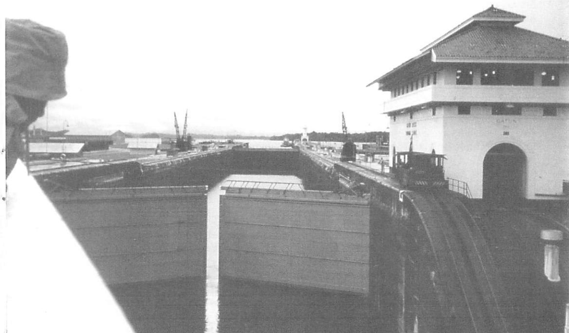
Lock on Panama Canal
